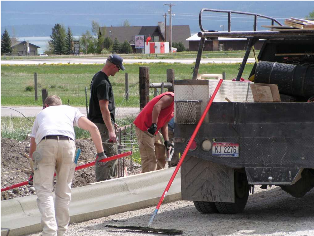
Curbs are being laid!
